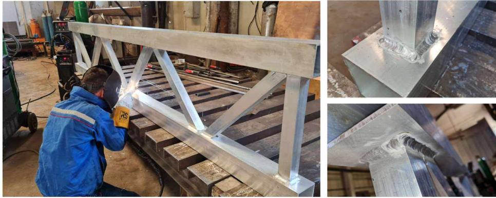
Fig.18: Welding of aluminium truss girders
